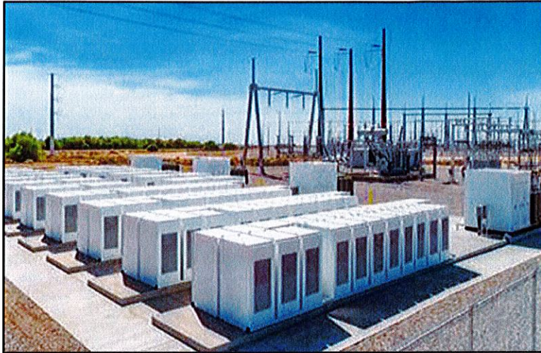
Figure 2b. Example self-contained energy storage system cabinet.
