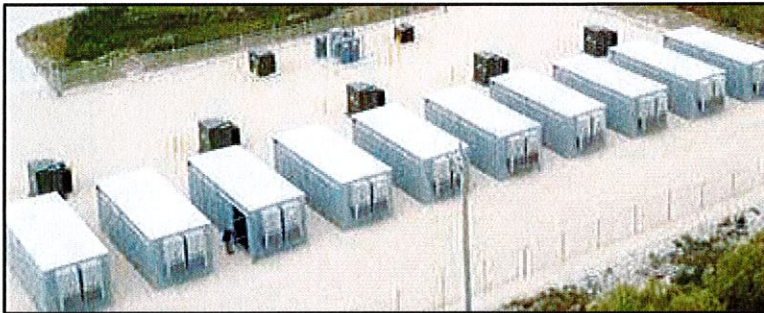
Figure 2c. Example self-contained energy storage system cabinet.
