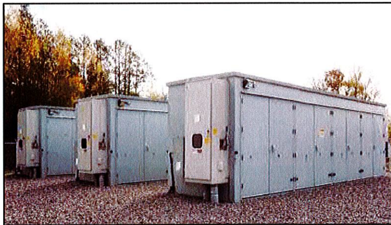
Figure 2a. Example self-contained energy storage system cabinet.
